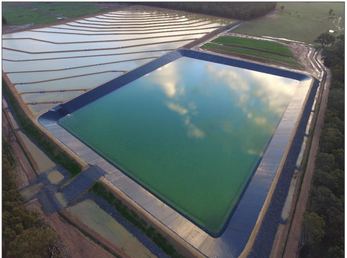
Figure 5.3: Ariel view of the Splitters Creek Evaporation Facility
