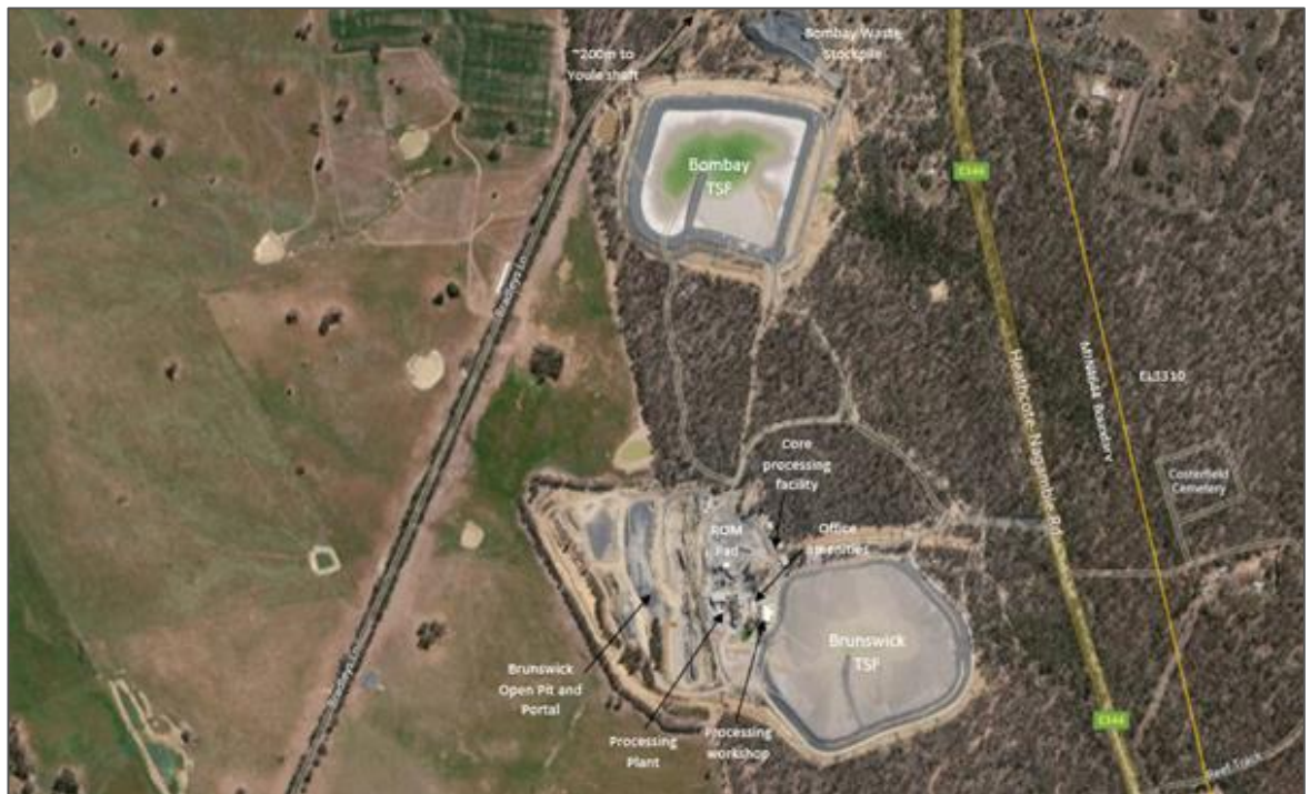
Figure 18.2: Brunswick Mine Site – aerial view
