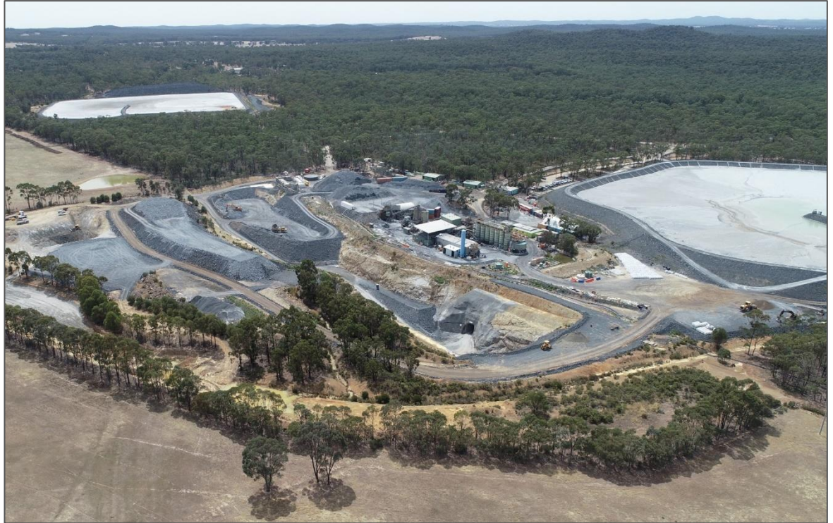
Figure 5.2: Aerial view of the Brunswick Complex with Brunswick Portal (middle of image), Brunswick Processing Plant, offices and tailing storage facilities
