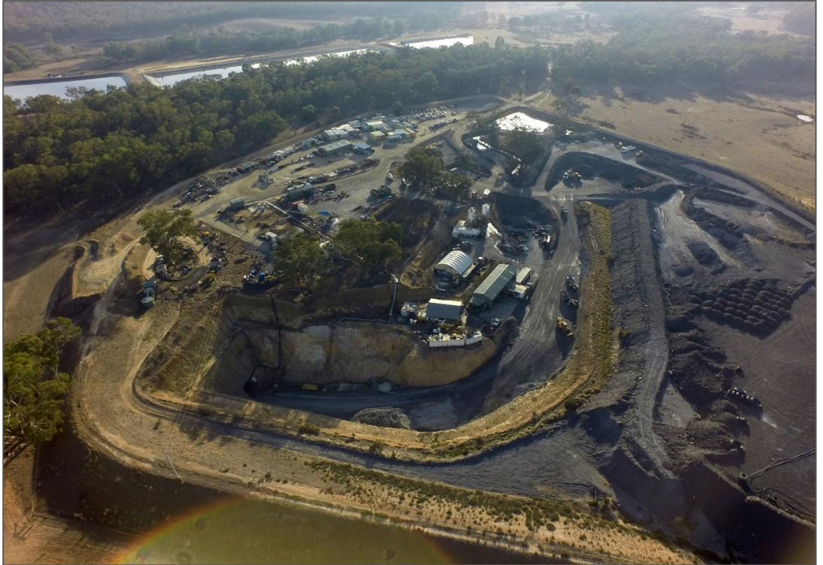
Figure 5.1: Augusta mine site with box cut, Augusta Portal (foreground), workshop, offices and holding dams
