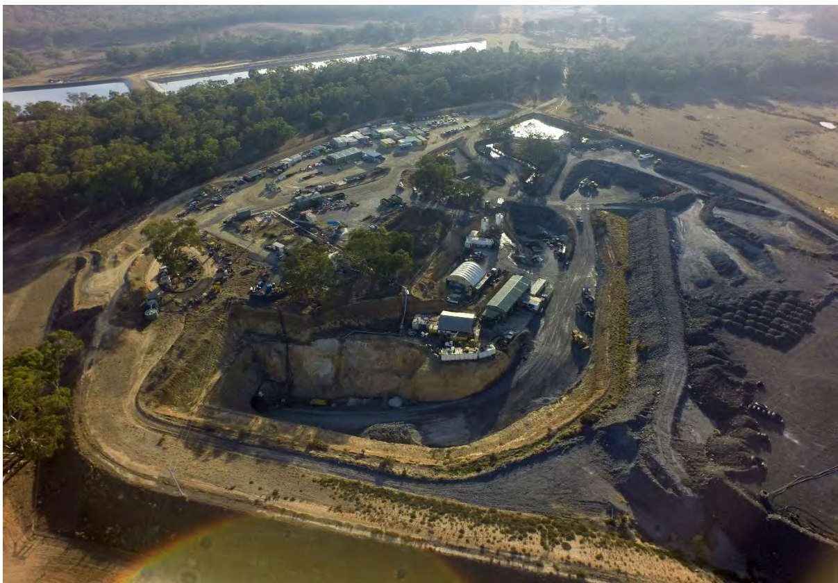
Figure 5-2: Augusta mine site with Boxcut, Augusta Portal (foreground), Workshop, Offices and Evaporation Dams
