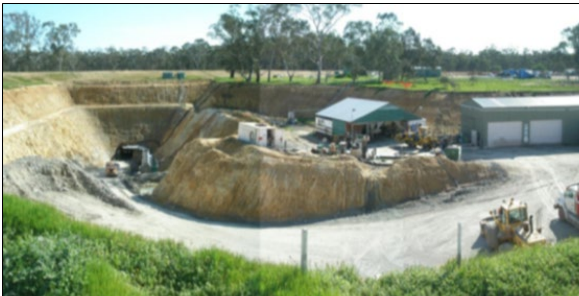
Figure 5-2: Augusta box-cut, portal and workshop
