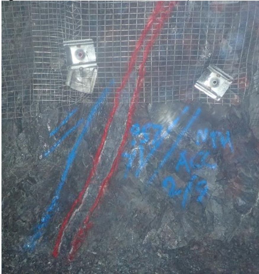
Figure 2: Youle Lode Face at the North Access, 957 Level
